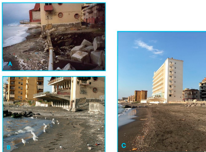
Figure 10. Recent evolution of the beach of the Miramare hotel. (A,B) the erosion processes had partially uncovered the foundations of the hotel structure. (C) weak progradation of the beach, now about 20 m wide.
