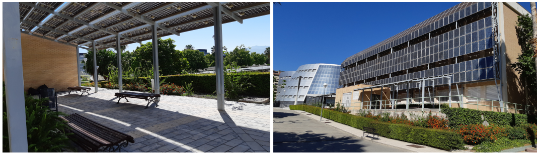
Figure 1. Two views of the photovoltaic (PV) generator of the UniVer Project. (a) PV pergola with semitransparent modules ; (b) East view of the PV facade.
