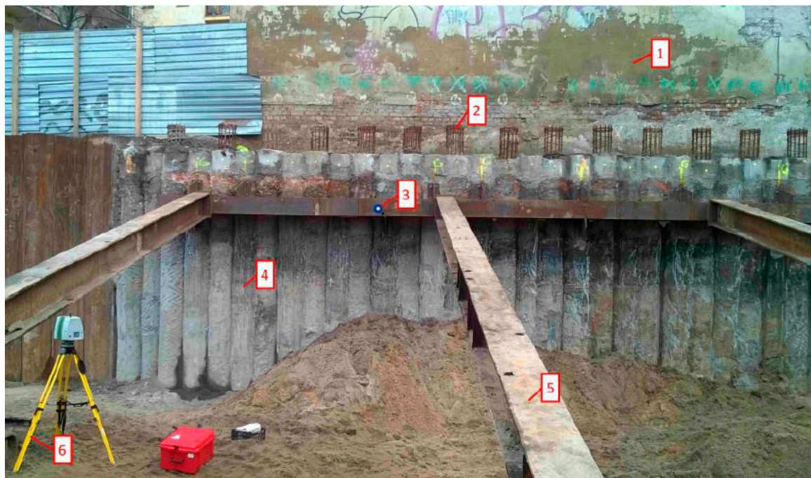
Figure 1. Protection of deep excavation by means of continuous flight auger (CFA) palisade: (1) the wall of the nearest existing building; (2) reinforcement cage; (3) special target used as the tie point for combining scanner positions; (4) palisade made of CFA piles; (5) steel strut; and (6) position of the laser scanner.
