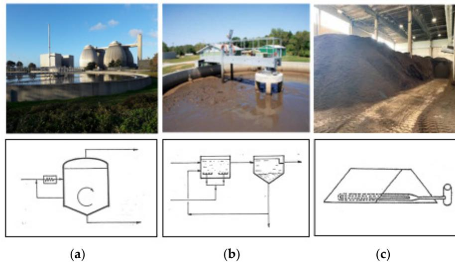
**Figure 4.** View of (a) anaerobic digestion, (b) aerobic stabilization, and (c) windrow composting.
