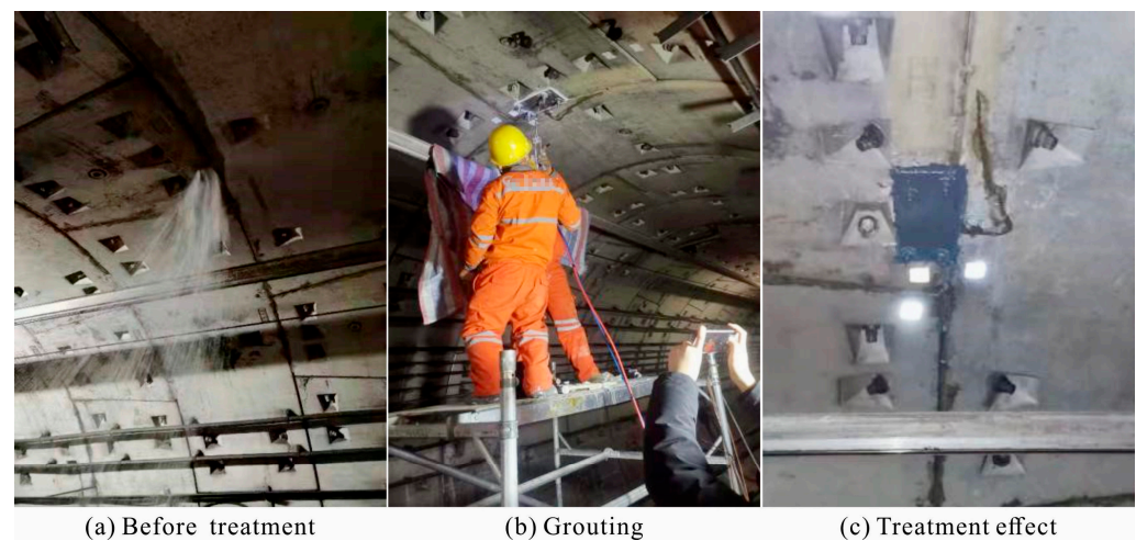
Figure 23. Sealing effect of LiB-AC grout.
