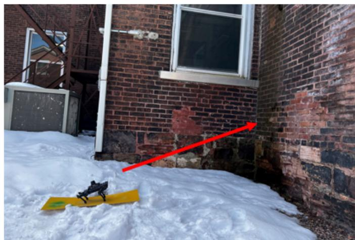
**Figure 9.** A tilting QRD aimed at the direction of the arrow to inspect the damaged area of the bulged wall using LiDAR.
