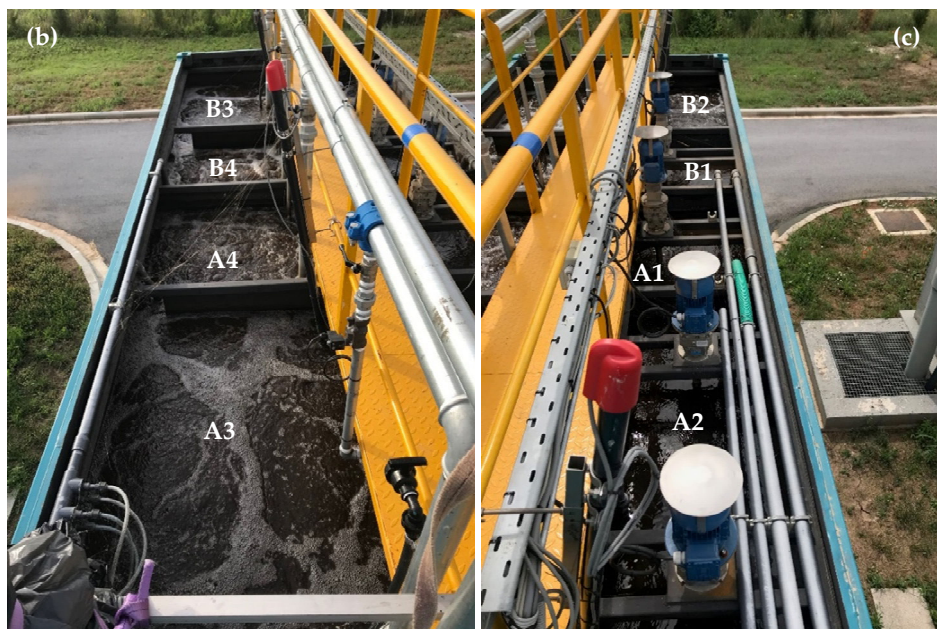
Figure S1. (a) Engine room equipment of the MBR, (b) Top-view of the MBR compartment's left side, (c) Top-view of the MBR compartment's right side (A1: Gentle stirring (de-aeration) tank of Control-MBR, A2: Denitrification tank of Control-MBR, A3: Aeration tank of Control-MBR, A4: Membrane tank of Control-MBR, B1: Denitrification tank of Filament-MBR, B2: Filament tank of Filament-MBR, B3: Aeration tank of Filament-MBR, B4: Membrane tank of Filament-MBR).
