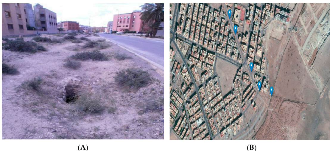
Figure 2. Khettara showing the Qanat shafts located in Marrakech city (A). Aerial view (B).
