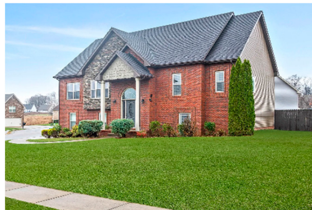
Figure 9. Case study 3: Two-story wood-frame residential building in Clarksville, Tennessee, damaged due to the tornado event in December 2023.
