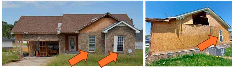
Figure 8. Case study 2: Intact glazing on windows and doors across the remaining areas of the building envelope outside the primary damage zone.
