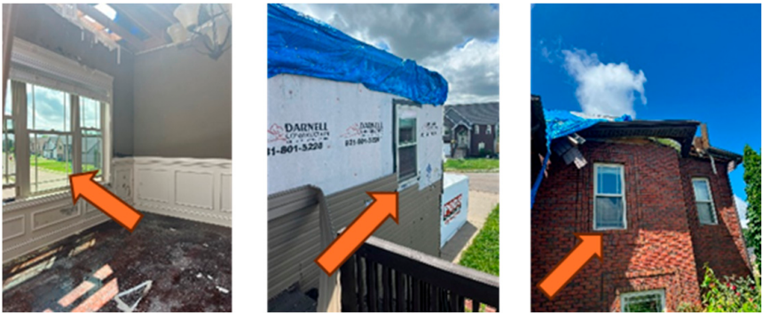
Figure 12. Case study 3: Intact window glazing on the building envelope.
