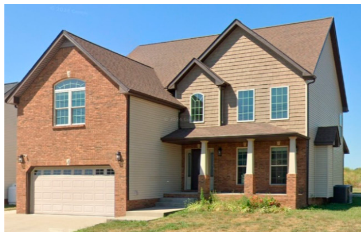
Figure 1. Case study 1: Two-story wood-frame residential building in Clarksville, TN.
