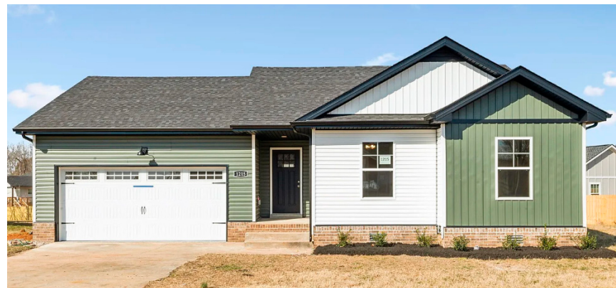
Figure 5. Case study 2: One-story wood-frame residential building in Clarksville, TN.
