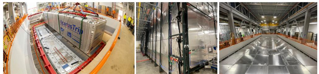
**Figure 2.** The east and west ICARUS cryostats were placed in the SBN Far Detector pit at Fermilab in August 2018 (left). A picture of the side CRT is shown (center). Installation of the top CRT horizontal modules was completed in December 2021 (right). The bottom CRT is not visible in these pictures.
