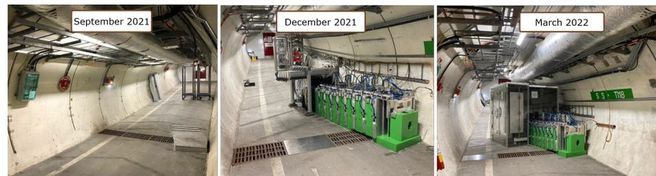
**Figure 3.** Detector installation in the TI18 tunnel.
