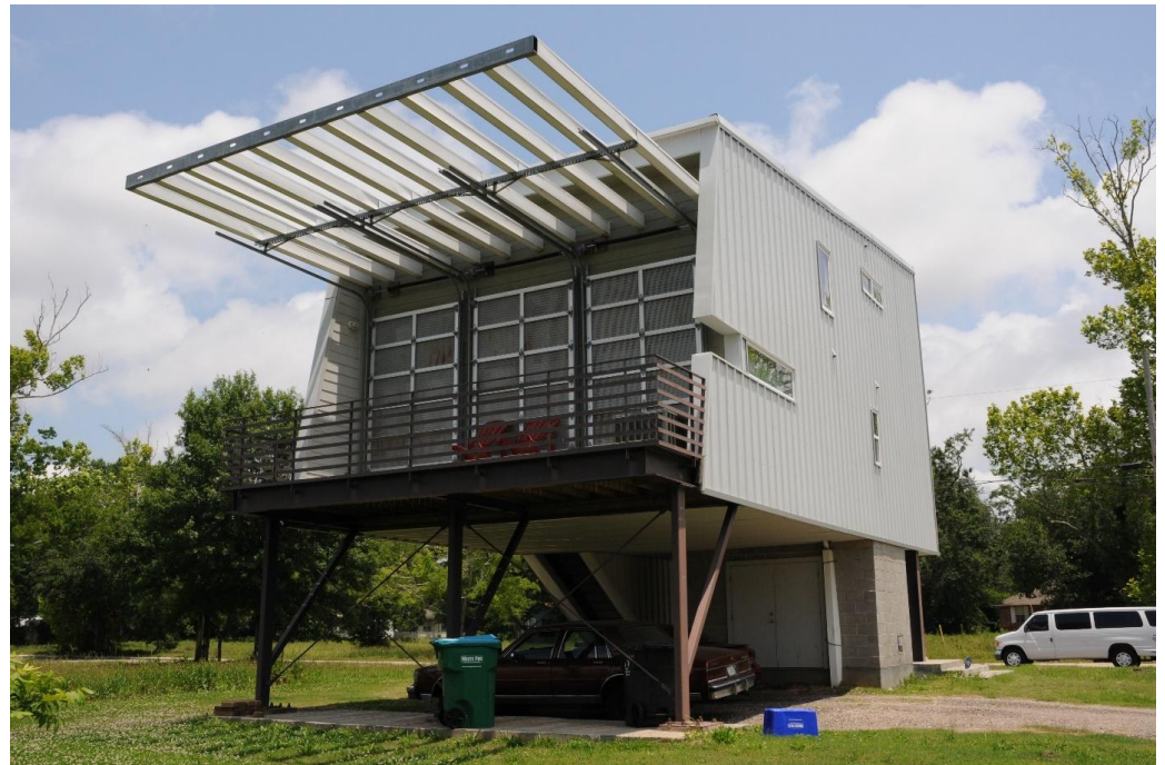
Figure 1. A house in Biloxi, USA, designed by Architect Marlon Blackwell after the 2005 Hurricane Katrina, which includes disaster-resilient features such as an elevated floor to mitigate floods and coastal storm surges, and a steel structure with bracings and metal cladding to resist wind impact (photo credit: Author).
