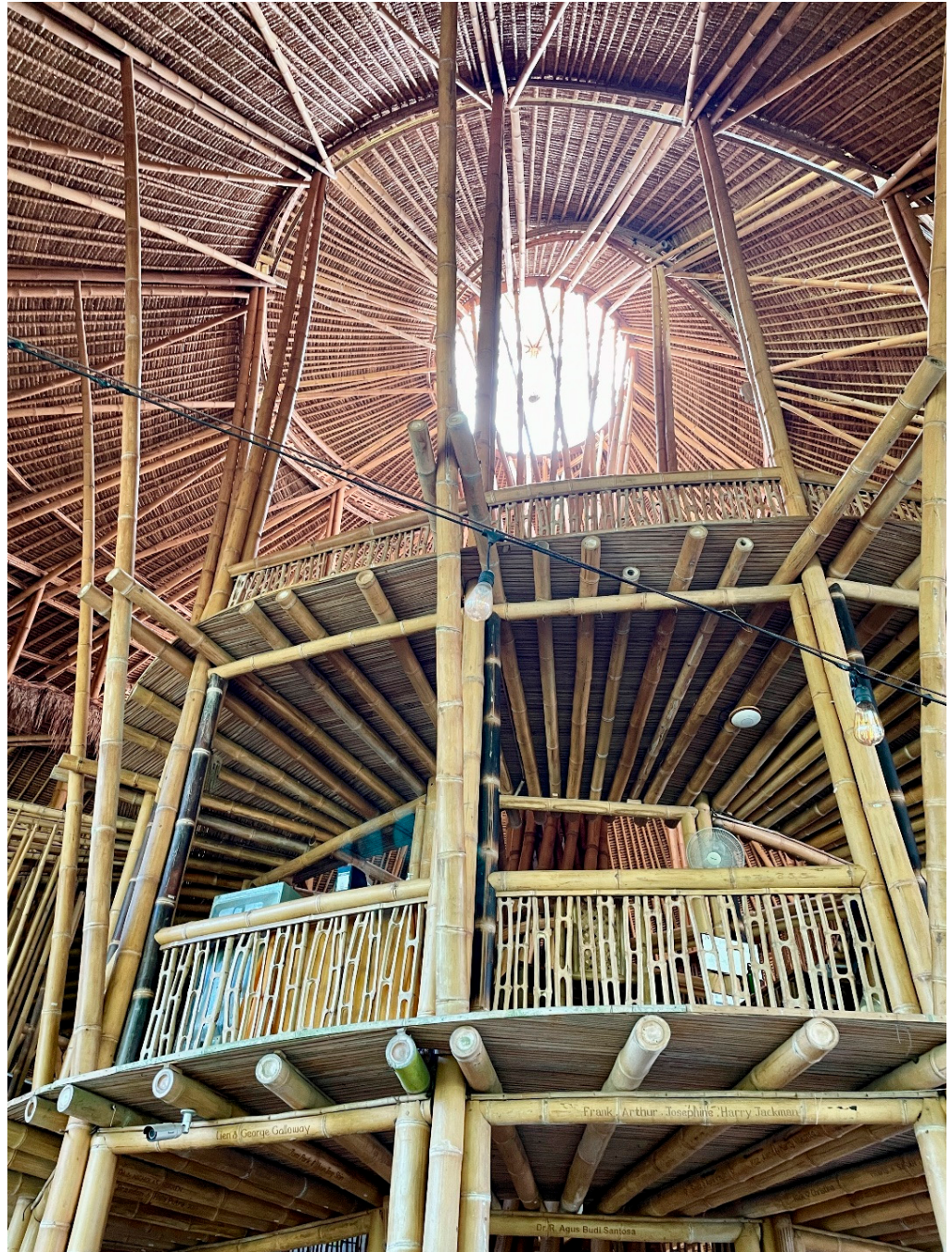
Figure 2. Towering bamboo columns supporting multi-level spaces of the Heart of the School. Photo: Fiona Gray.
