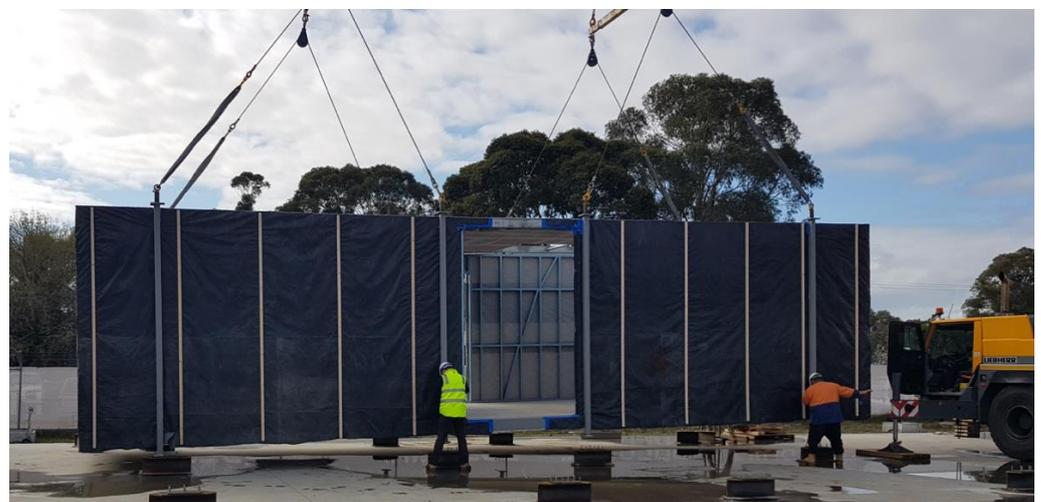
**Figure 7.** A partly finished structural module being lifted into place using a top-lift method where the lifting mechanism is properly connected to full-length structural columns.
