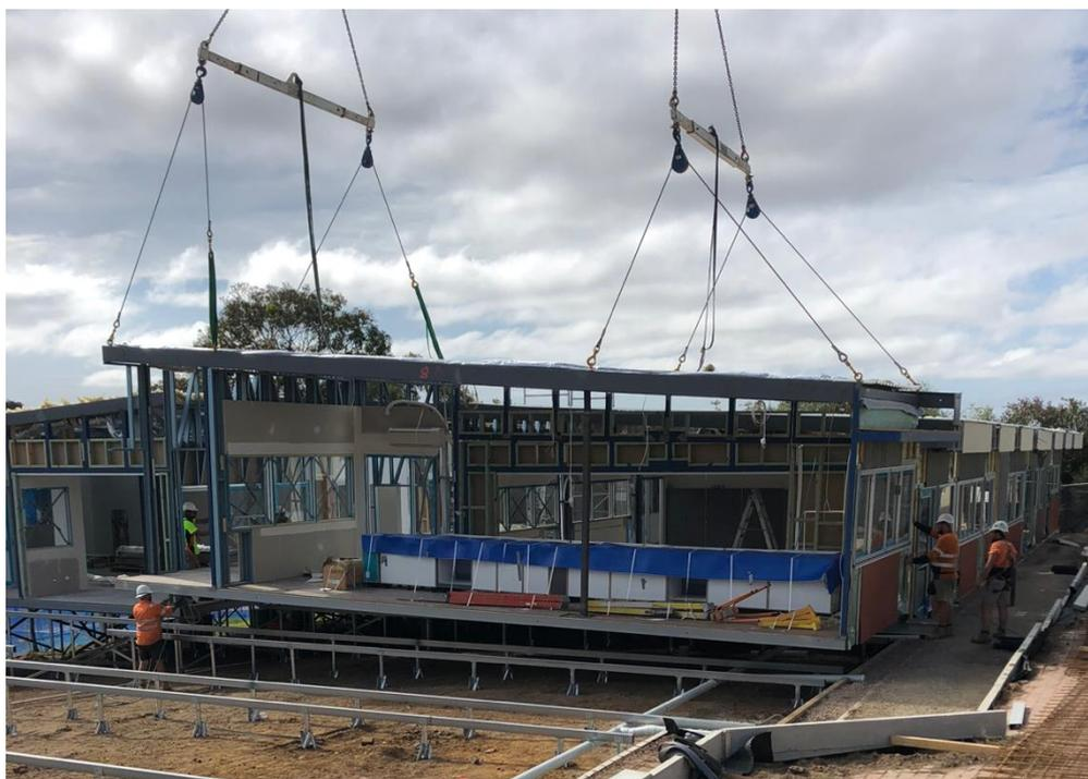
**Figure 18.** A partially finished modular unit being installed on top of a prefab foundation (driven piles with a base plate and steel bearers on top).
