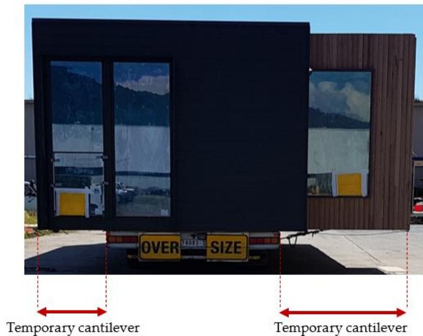
**Figure 5.** Temporary support conditions—An example of a situation where cantilevers which would not be there in the final state of a structure are imposed on a module during transportation.
