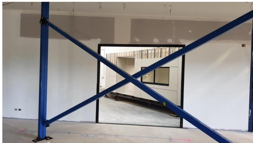
**Figure 4.** A temporary cross bracing applied between two temporary columns in a prefabricated volumetric module (all to be removed after installation).
