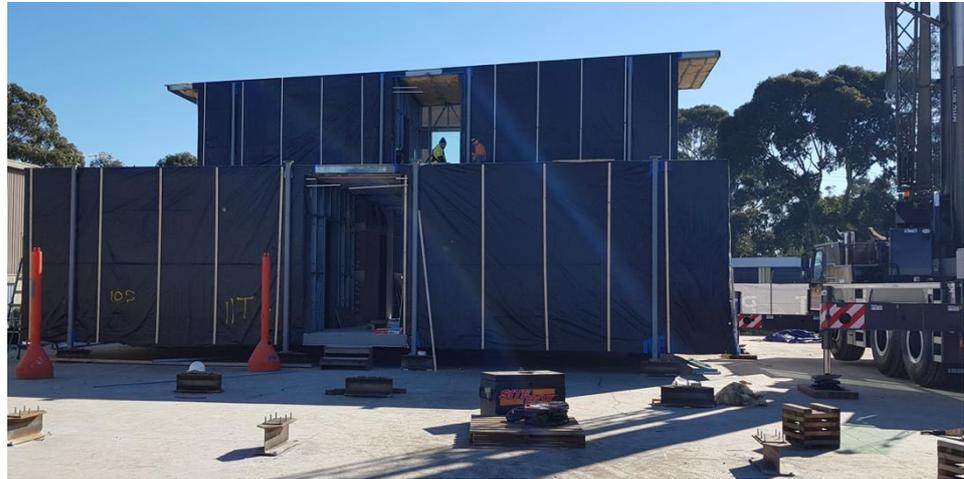
**Figure 16.** Example of a full-scale prototype carried out within the manufacturing facility of a prefab builder for a double storey-steel modular building to check issues in buildability and installation sequence.
