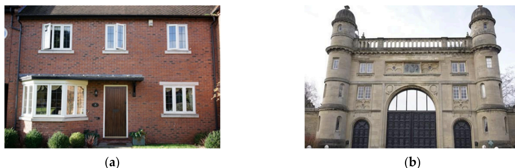
Figure 3. (a) Dunrobin House, Warwickshire, UK; (b) Lenton Lodge Gatehouse, Nottinghamshire, UK.
