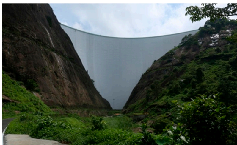
Figure 30. White reflective coating applied on the entire intrados face of the dam.
