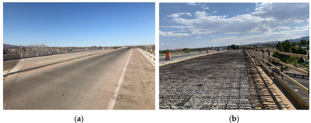
**Figure 3.** Bridge no. 7032—(a) before and (b) after initial deck removal.
