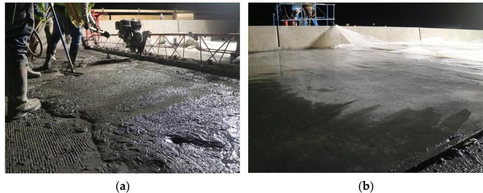
**Figure 6.** UHPC overlay (a) placement and (b) finish.
