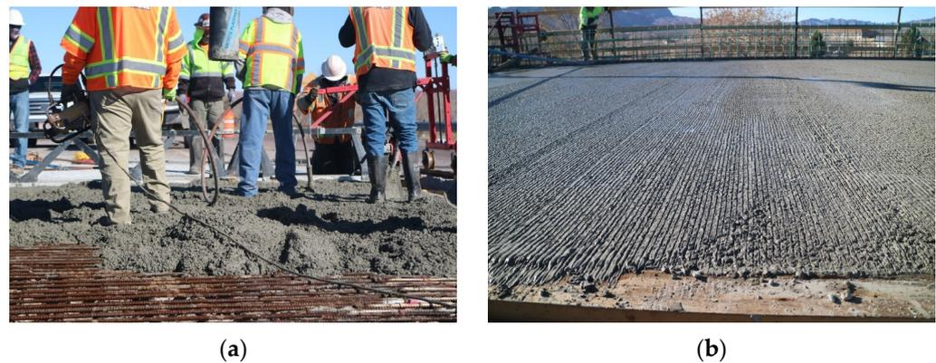
**Figure 5.** High-performance deck (HPD) (a) placement and (b) finish.
