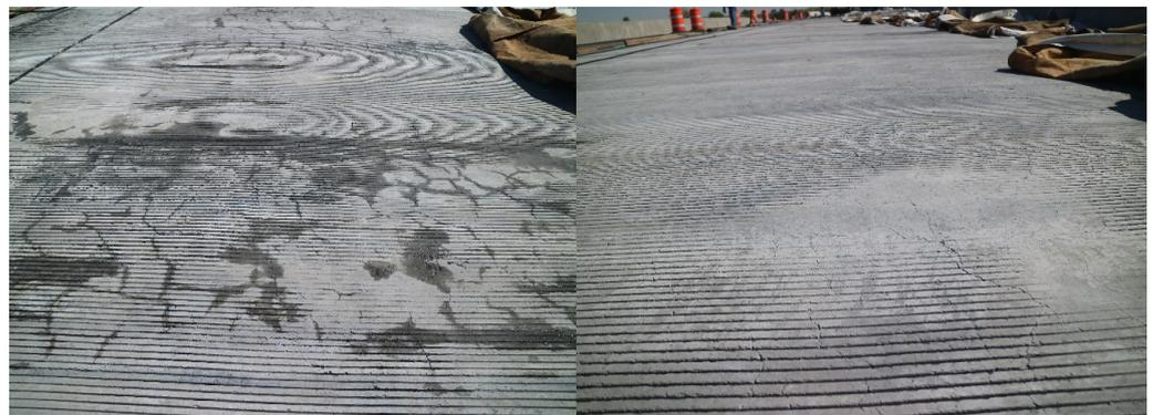
**Figure 7.** Overlay cracking from Production Placement 1.
