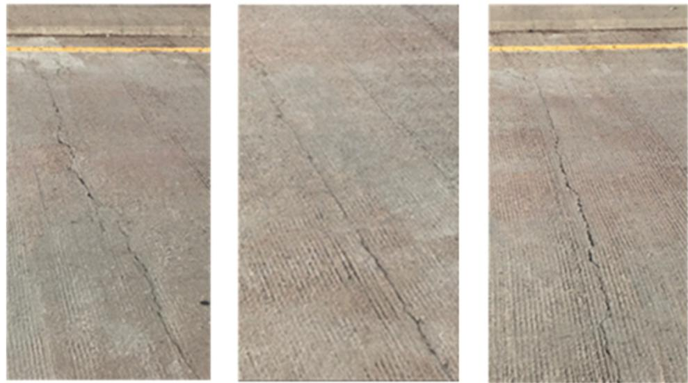
**Figure 2.** Transverse cracks within negative moment regions of existing concrete deck.
