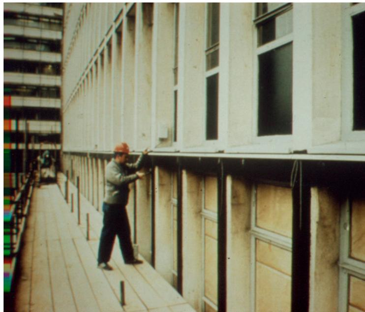
**Figure 6.** Conductive coating being applied to reinforced concrete columns and beams on a building in London, England. Reprinted from Ref. [1] with permission. Copyright 2007 Taylor and Francis.
