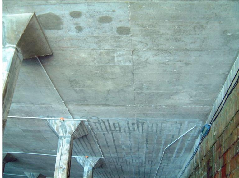
**Figure 4.** Ribbon anodes in the soffit of a reinforced concrete jetty in Jersey, UK.
