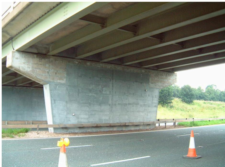
**Figure 7.** Arc-sprayed zinc anode applied to the substructure of a highway bridge in the north of England. Reprinted from Ref. [1] with permission. Copyright 2007 Taylor and Francis.
