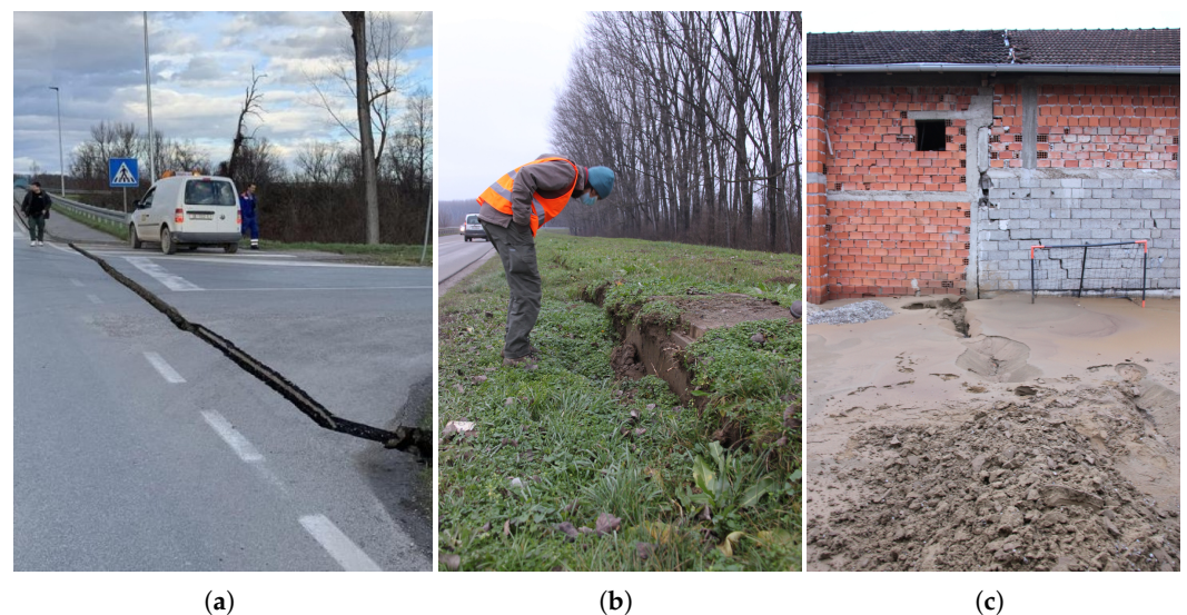
Figure 2. Manifestations and consequences of liquefaction-induced lateral spreading at Brest Pokupski following the 2020 Petrinja earthquake: (a) damage to the bridge crossing and adjacent roadway infrastructure caused by permanent ground deformation (photograph: index.hr portal), (b) longitudinal cracking and deformation of the flood protection levee, and (c) sand ejecta and surface evidence of liquefaction documented in the Brest Pokupski site.
