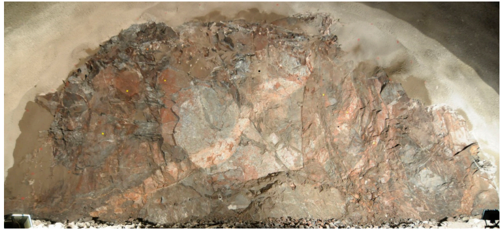
Figure 2. Tunnel face with blocky monzogranite rock. (photo by the author with permission from PURAM).
