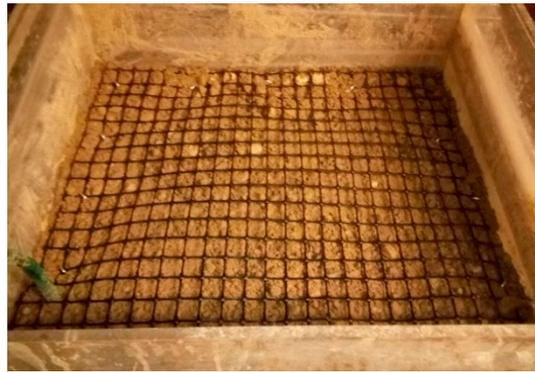
Figure 17. Geogrid installation in HGRS section.
