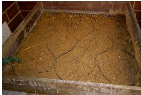
Figure 18. Geocell installation in HGRS section.
