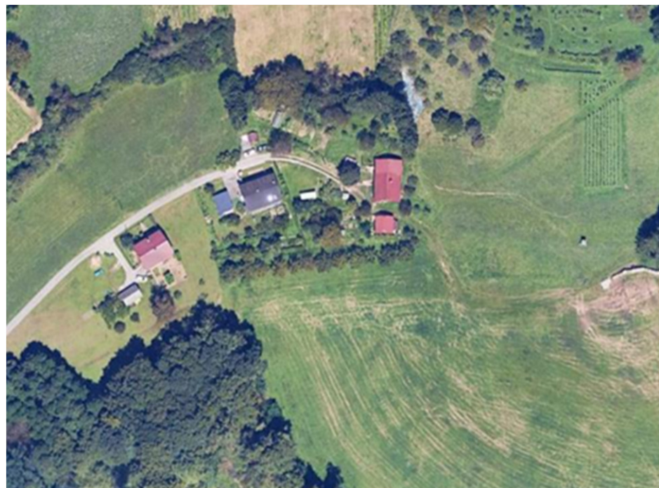
Figure 10. Overview of the landslide area.
