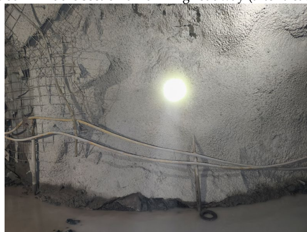
(d) Entrance of rock drilling roadway at 0-5-6 mining site in the middle section of –1020 m (after treatment)
