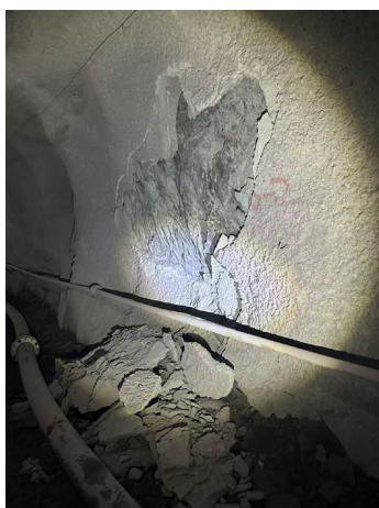
(a) –960 m middle section 0–26 filling roadway
