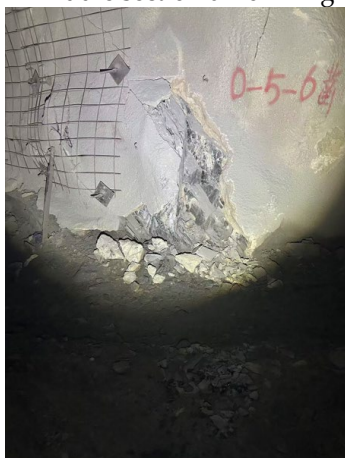
(c) Entrance of rock drilling roadway at 0-5-6 mining site in the middle section of –1020 m
