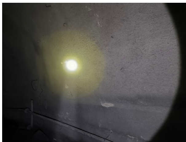
(b) –960 m middle section 0–26 filling roadway (after treatment)
