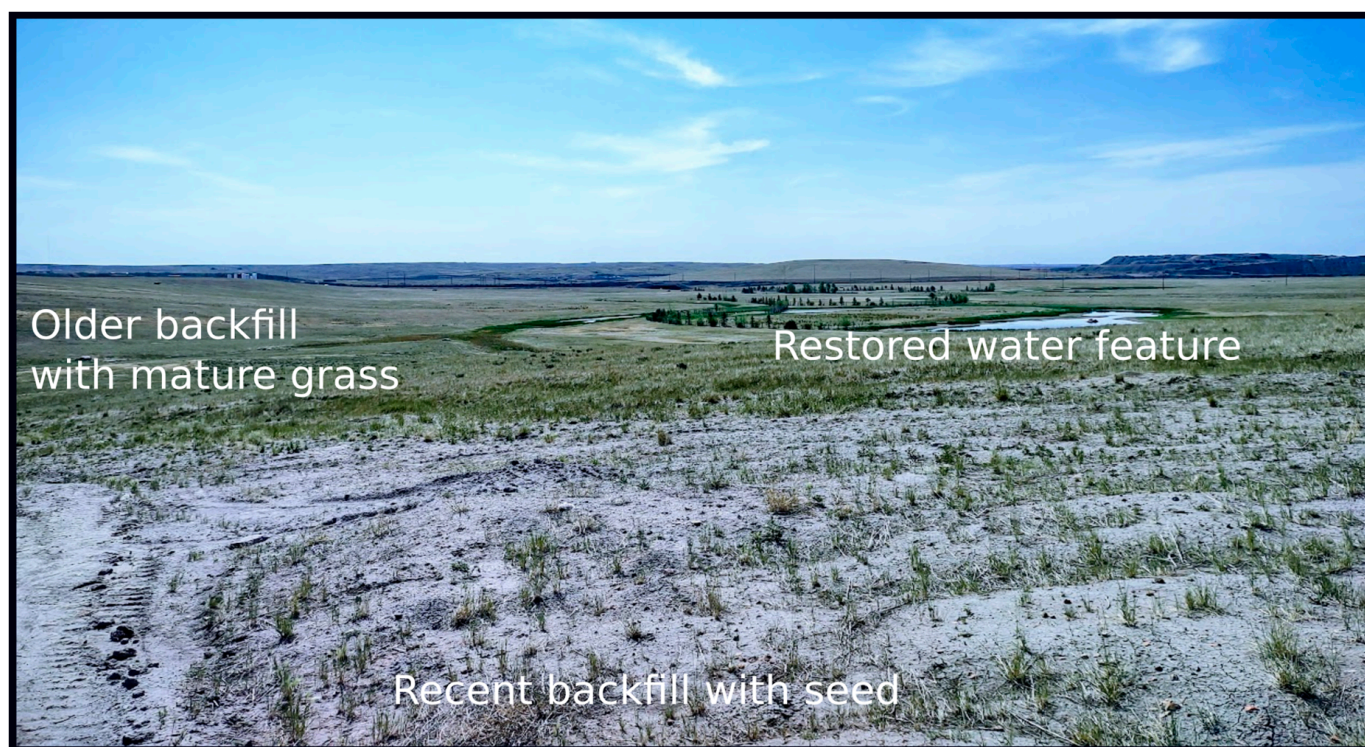
Figure 4. Reconstructed landscape adjacent to the active Cordero Rojo Mine, Powder River Basin, Wyoming, USA. The coal pit has been filled with waste rock (backfill), graded, and covered with seeded topsoil along with reconstruction of water features.
