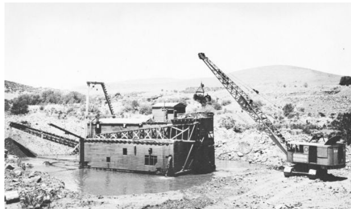
Figure 13. Dredge operated in Lynx Creek by the Calari dredging Co., 1933. Capacity of 100 cubic yards per hour [59].
