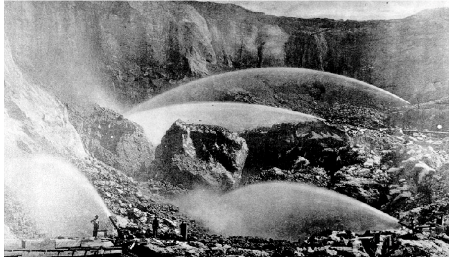
Figure 8. Hydraulic mining at Malakoff Diggings (Historic photograph taken by Watkins) [45].
