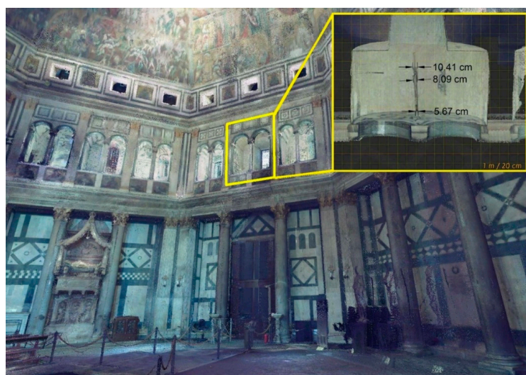
Figure 6. Scanning data highlighting the dimensions of a crack above the north door of the Baptistery di San Giovanni in Florence. Source: [29]. Figure 12, page 257.
