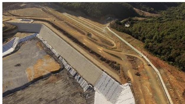
**Figure 9.** Downstream embankment construction.
