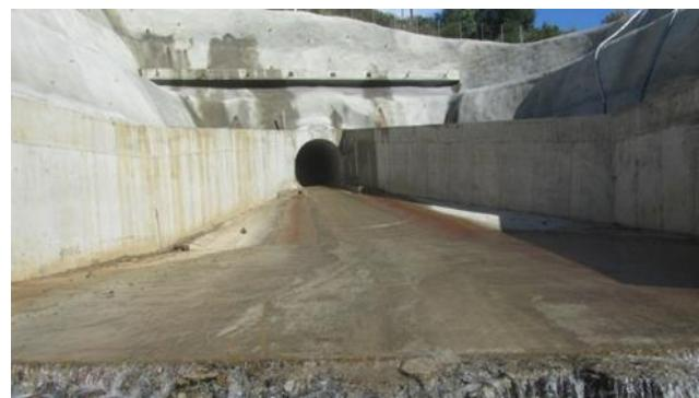
**Figure 3.** Diversion tunnel exit portal.
