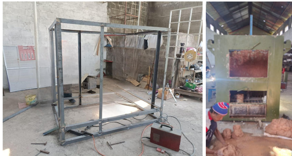
Figure 3. Construction of Incinerator and installation of refractory stone wall.
