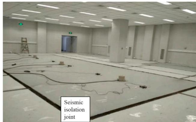
Figure 1. Site drawing of vibration isolation platform.
