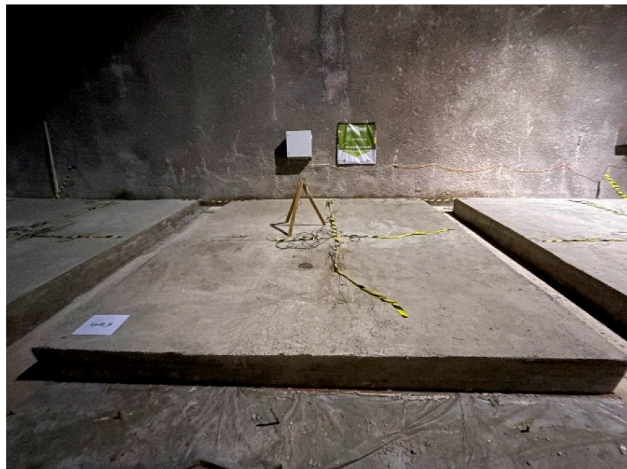
Figure 1. The three large, reinforced test slabs were cast and monitored on site.
