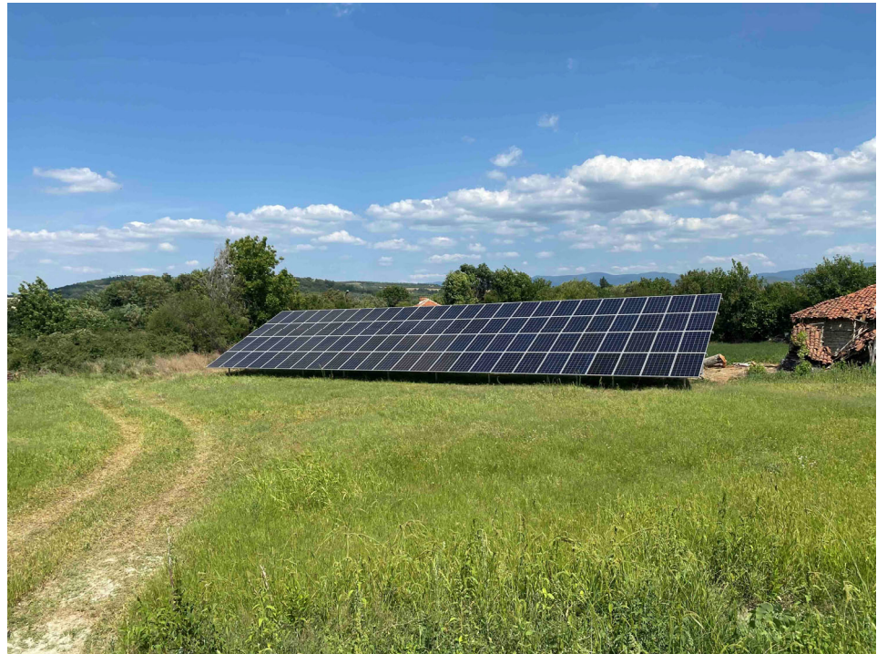
Figure 7. Optimal installation. Note that proper string configurations allow for slight degradation during ground foliage periods.
