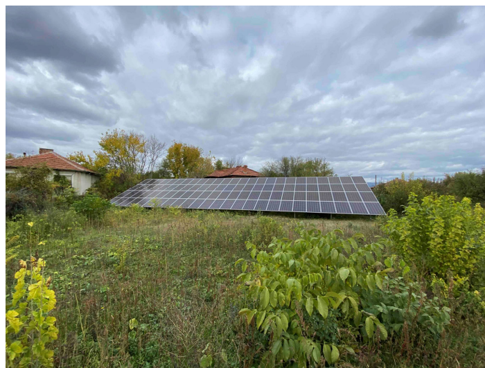
Figure 8. Optimal installation but poor maintenance of growth around it.
