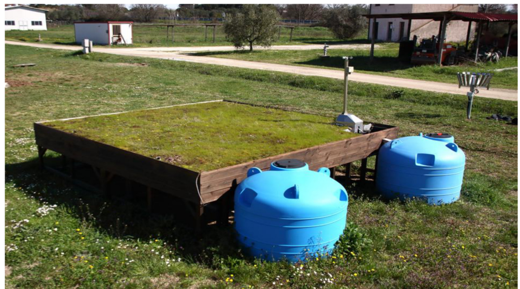
Figure 1. The investigated Polder Roof.
