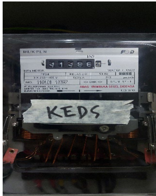
Figure 1. Sample image of an analog electricity meter from the Fuji Dharma brand to be annotated with digit labels (Digit-kWh).
