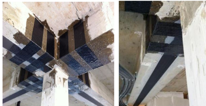
Figure 1. Examples of external strengthening of RC members.
