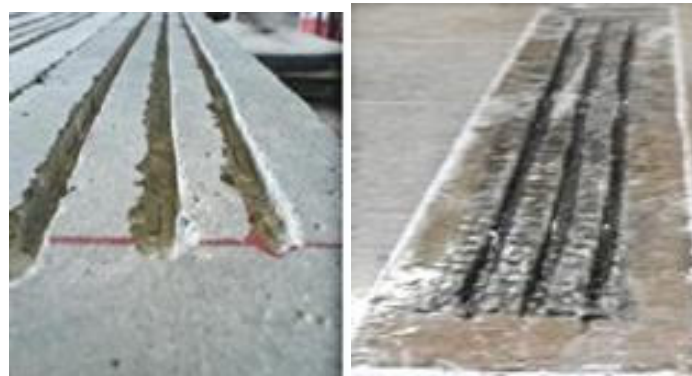
Figure 4. Reinforcement of the exterior using the EBRIGI technique (Mostofinejad and Shameli, 2013) [12].
