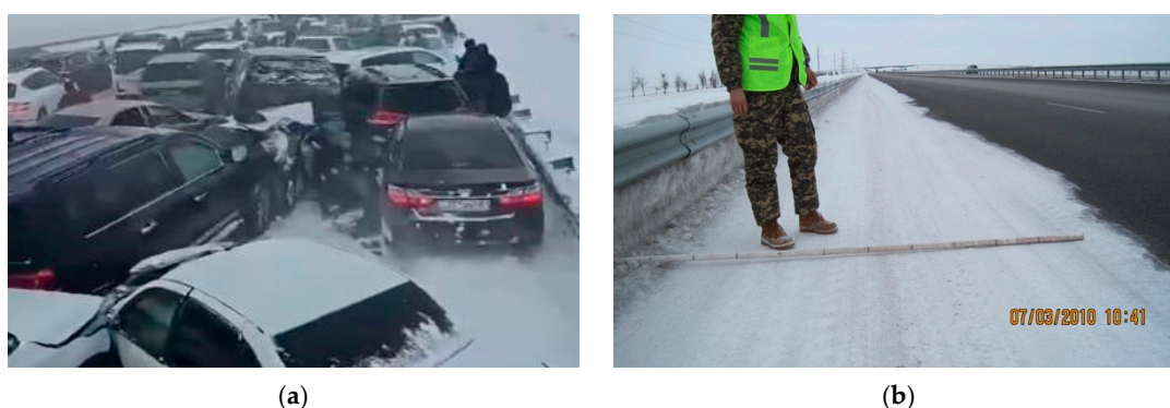
Figure 1. Mass traffic accident on the 104 km section of the Astana–Shchuchinsk highway (a) and snow–ice compaction with uncleared edge zones of the carriageway (b).
