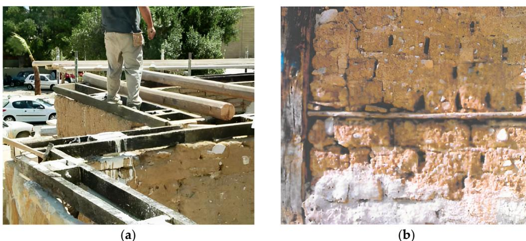
**Figure 1.** (a) Installation of wooden ring beams during construction [27]; (b) position of wooden ring beams [26].
