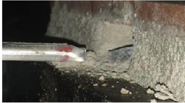
**Figure 6.** Example of tie connection failure mode observed for the tie type under consideration.
