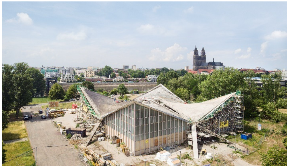
Figure 5. Strengthening process of the hypar shell in Magdeburg with CRC from 2020. (Photo: M. Bredt).
