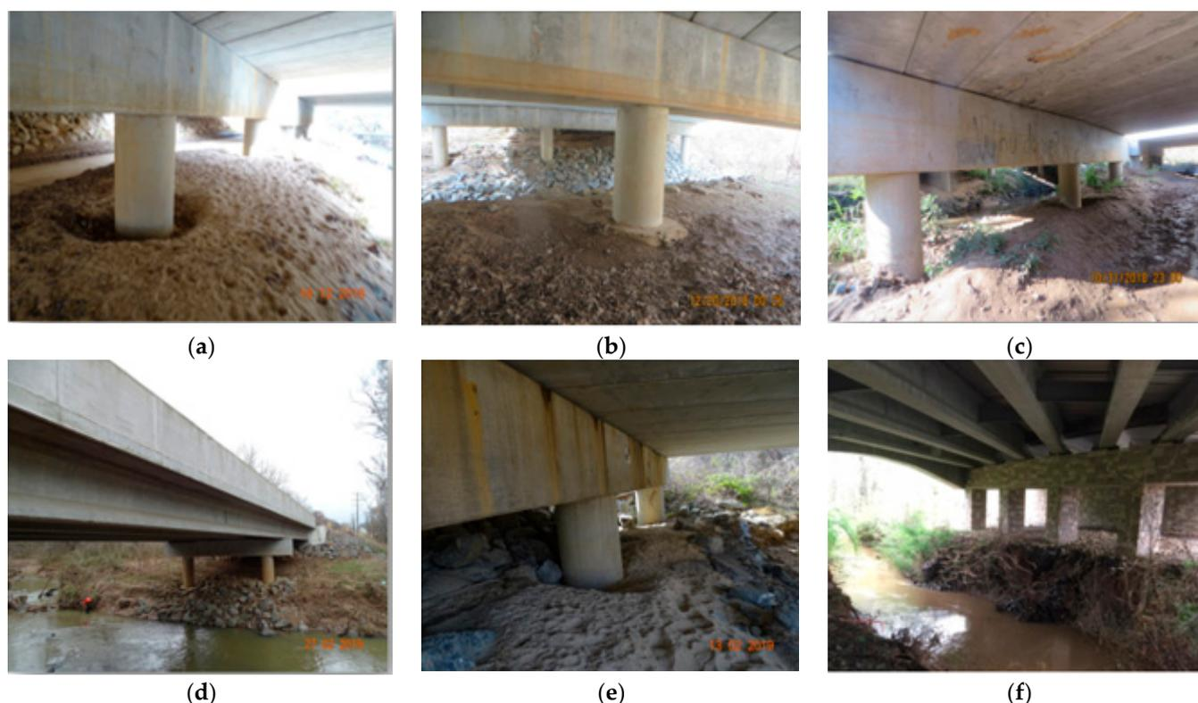
**Figure 1.** Examples of bridges with piers-on-bank and experiencing scour (a) Rocky River; (b) Mallard Creek; (c) Pharr mill; (d) Blackwood Creek; (e) Rankin Lake; (f) Toby Creek.
