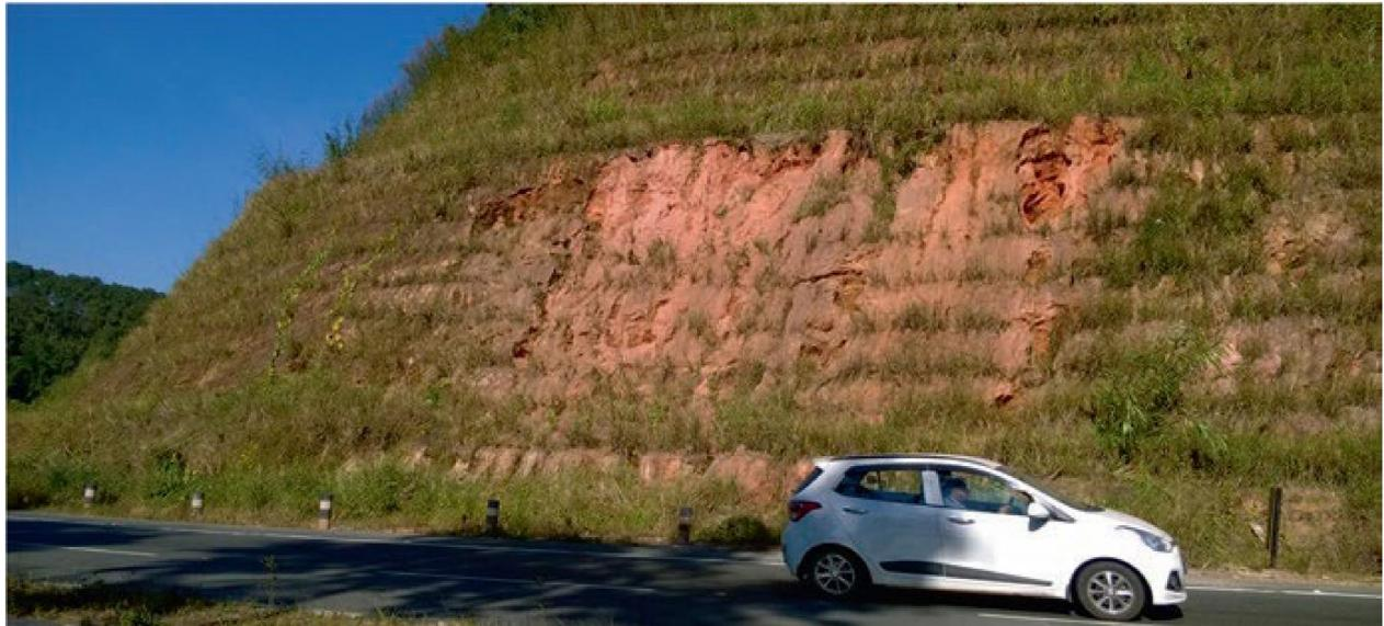
**Figure 2.** Vetiver grass stabilizing a cut slope along the Guwahati–Shillong National Highway, Meghalaya State, India as of July 2015 [20].
