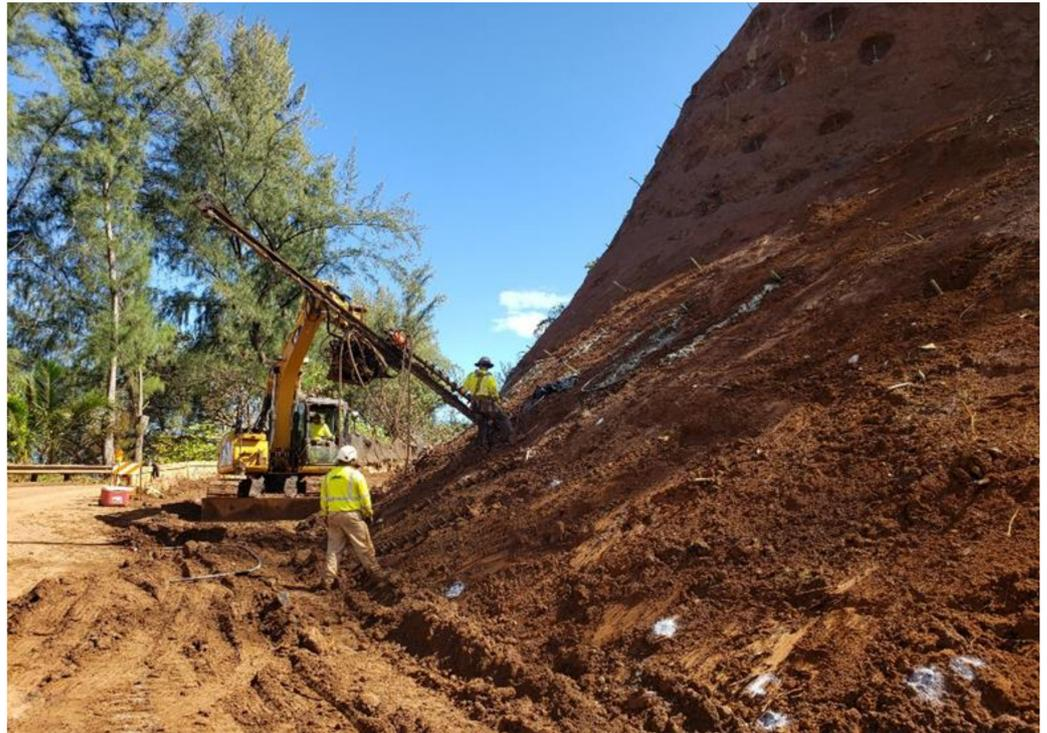
**Figure 4.** Landslide stabilization with metal soil nails. Source: Authors.
