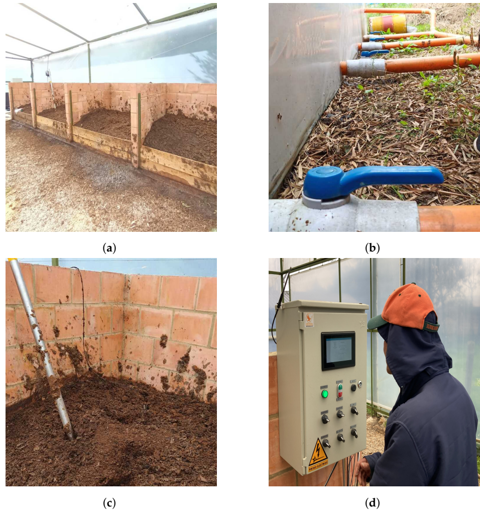
Figure 3. Commissioning of the automated composting plant with forced aeration: (a) cubicles loaded with chicken manure, (b) forced aeration techniques, (c) sensor implementation in the biopile, (d) plant verification and commissioning.
