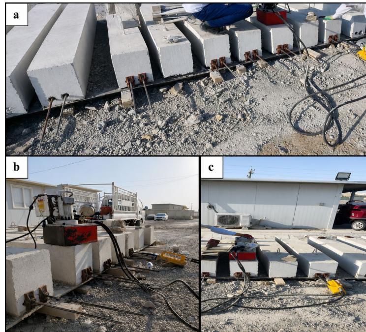
Figure 5. Prestressing operations: (a) tendon preparation before stressing, and (b,c) application of prestressing force using a hydraulic jack system.
