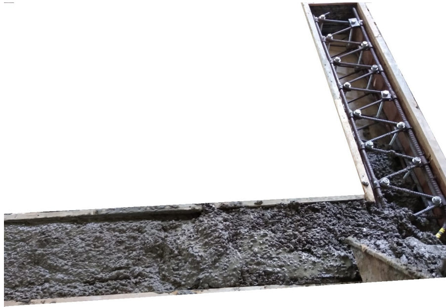
Figure 5. Concrete casting of the proposed specimen reinforced with a rebar truss system.
