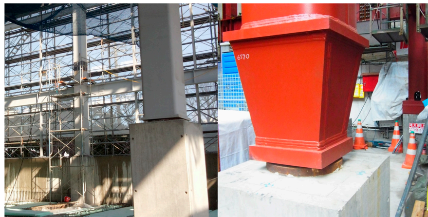
Figure 2. Industrial applications of MSP (mid-story pin) systems.
