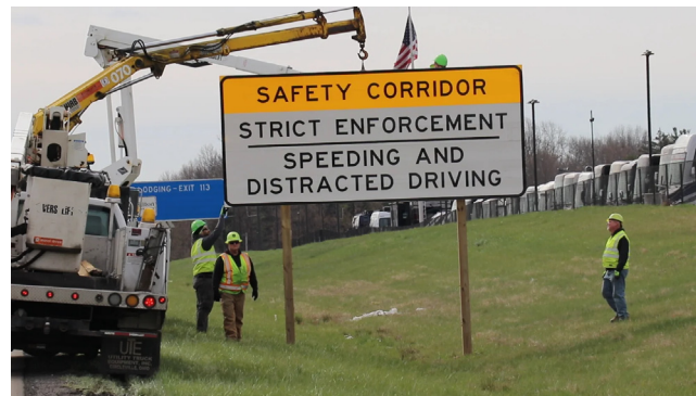
Figure 2. Increased signage at a distracted driving and speeding safety corridor in Ohio [20].
