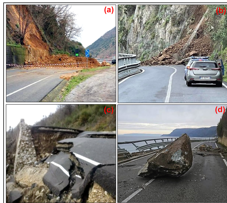
Figure 10. Photos of representative landslides affecting roads across the study area. (a) Earth slide blocking the entire carriageway of a section of the SP road; (b) rock-slide obstructing the SS18 road; (c) scarp of a complex landslide involving the SC road; (d) rock fall triggered on a steep slope and affecting the SS18 roadway.
