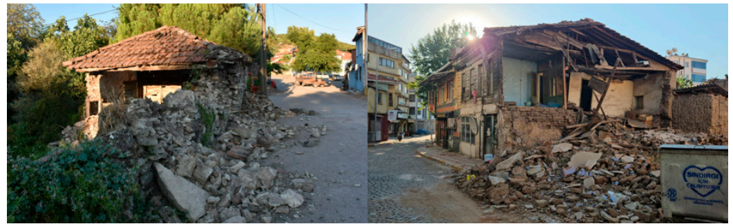
Figure 13. Out-of-plane wall damage samples.
