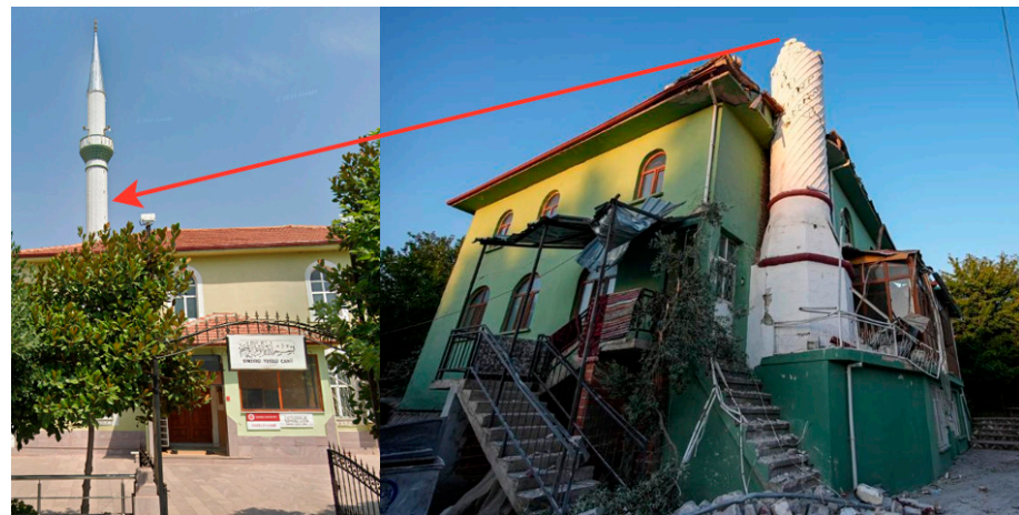
Figure 12. Pre and post-earthquake images of the minaret.
