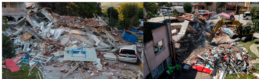
Figure 10. Post-earthquake images of the RC structure that totally collapsed.
