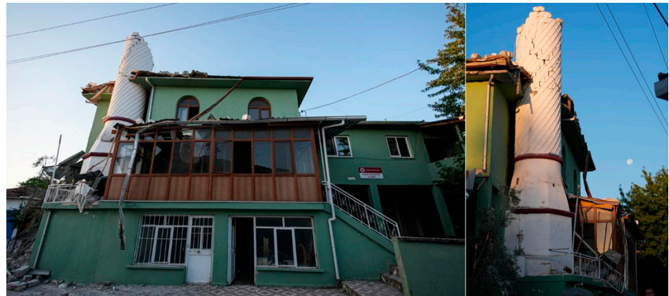
Figure 11. Front and side views of a minaret after the Balıkesir earthquake, showing damage to the minaret and partial collapse of the mosque.
