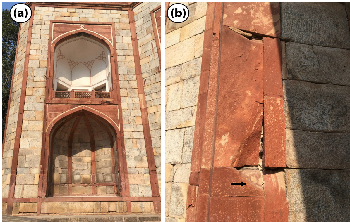
Figure 6. (a) Damage to the entrance gate of Humayun's Tomb; (b) the reddish stone block fractured at the corner due to the repeated shaking, detail indicated by black arrow.
