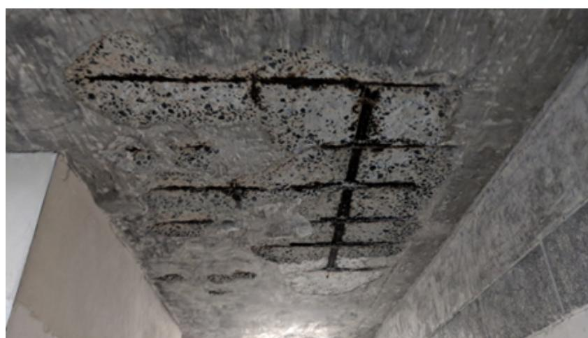
**Figure 3.** Example of concrete carbonation and corroded steel reinforcement.
