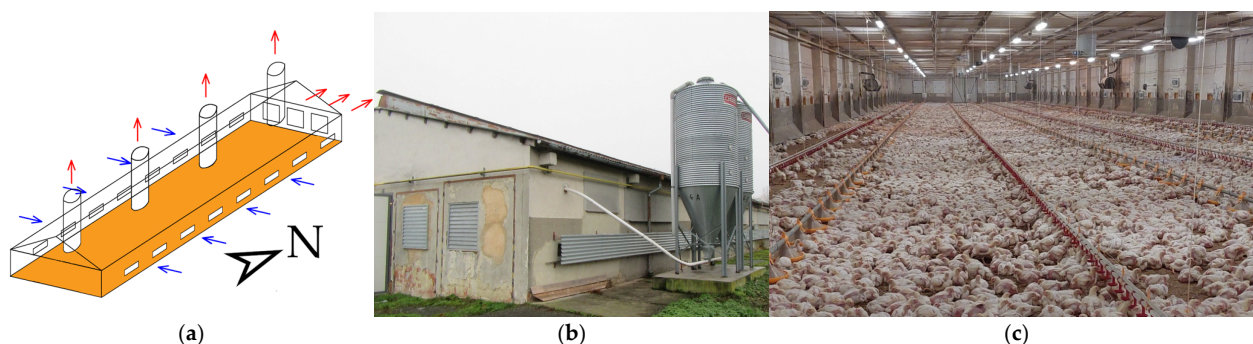
Figure 2. Hall H3: (a) air supply and exhaust; (b) external view; (c) internal view.
